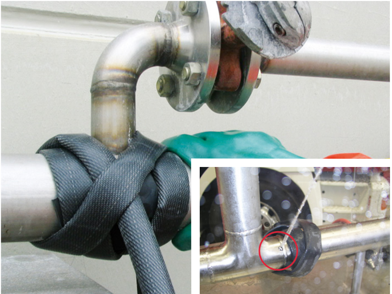
Precise-fitting sealing of difficult leaks
